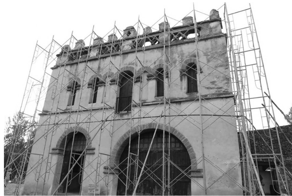
The renovation works of the Fasilides Castle
