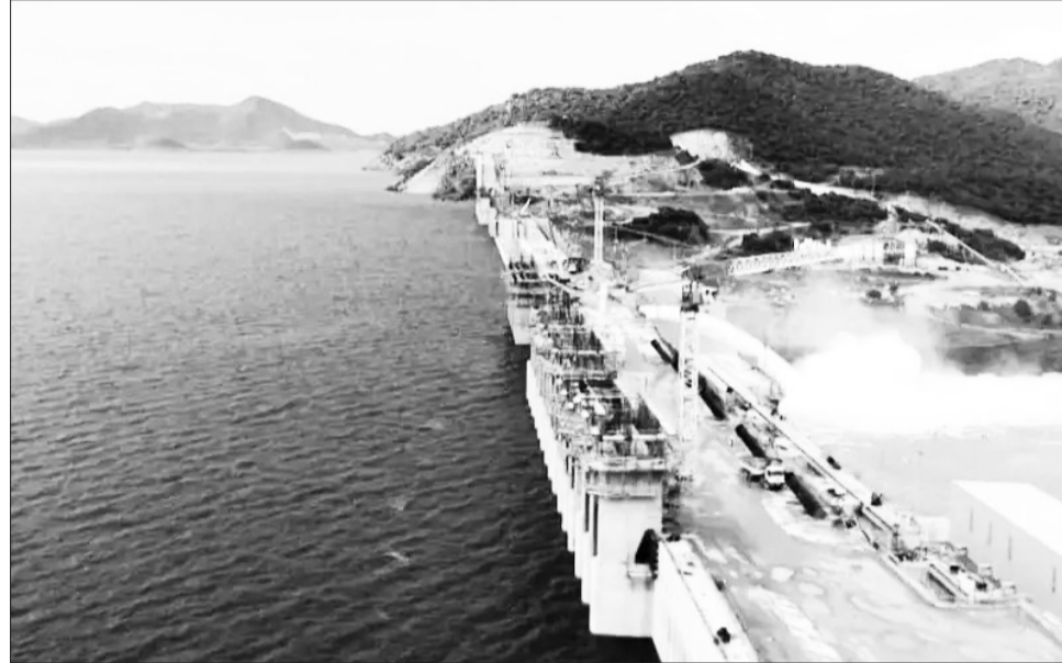
Abbay Dam near completion
