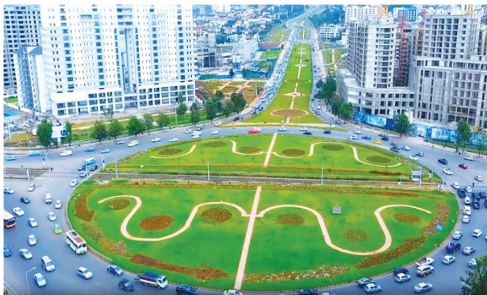
Partial view of Addis Ababa road corridor development
