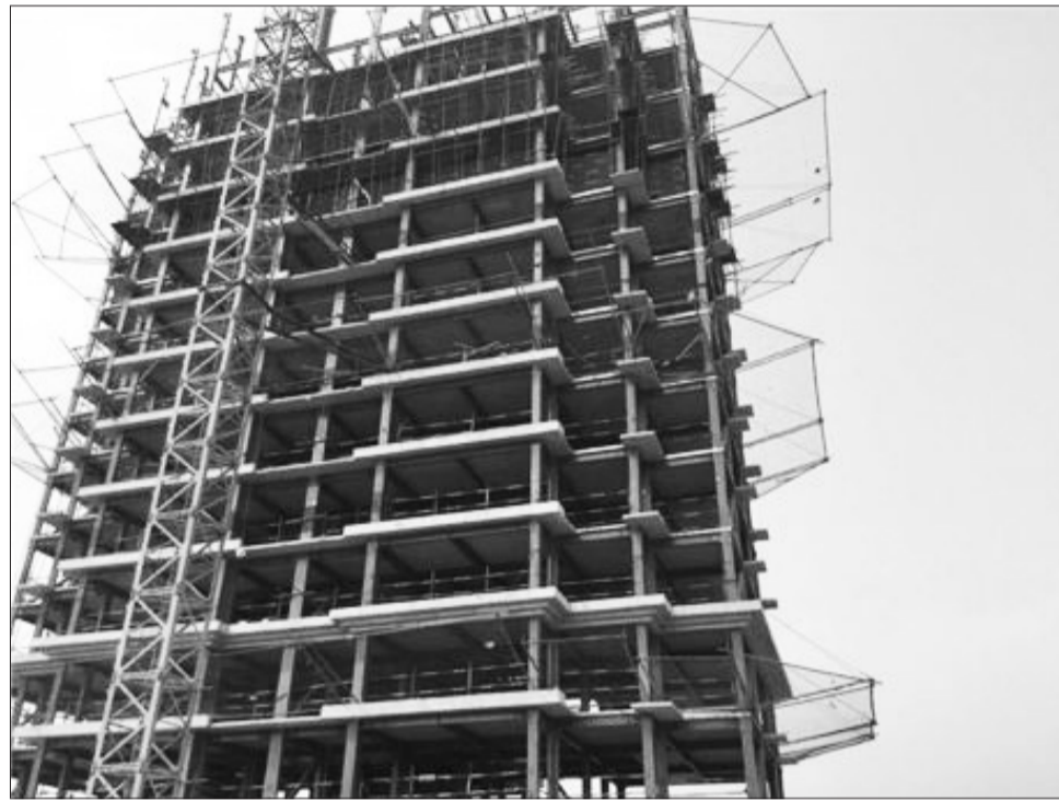
Some construction works delay due to shortage of inputs
