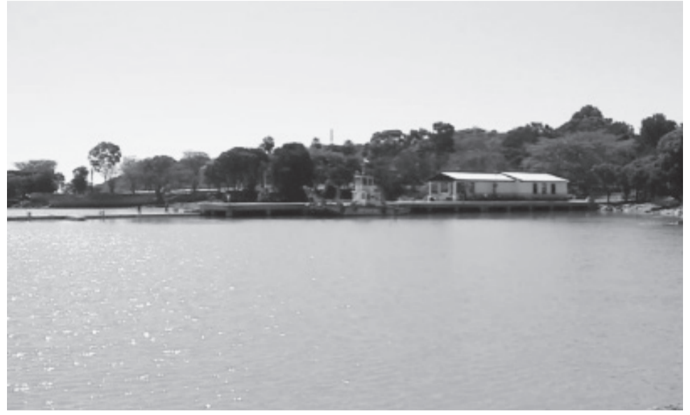
Gorgora Project nearing completion
